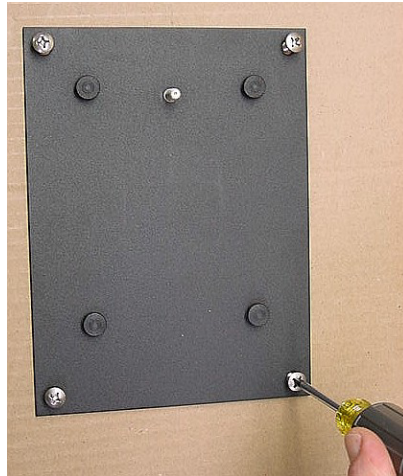
Figure 8. Secure mounting plate to wall.
