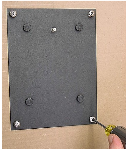
Figure 8. Secure mounting plate to wall.
